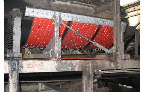
Coal harbour - 3.200 tons per hour 1600 Belt - speed 3,2 m / second
